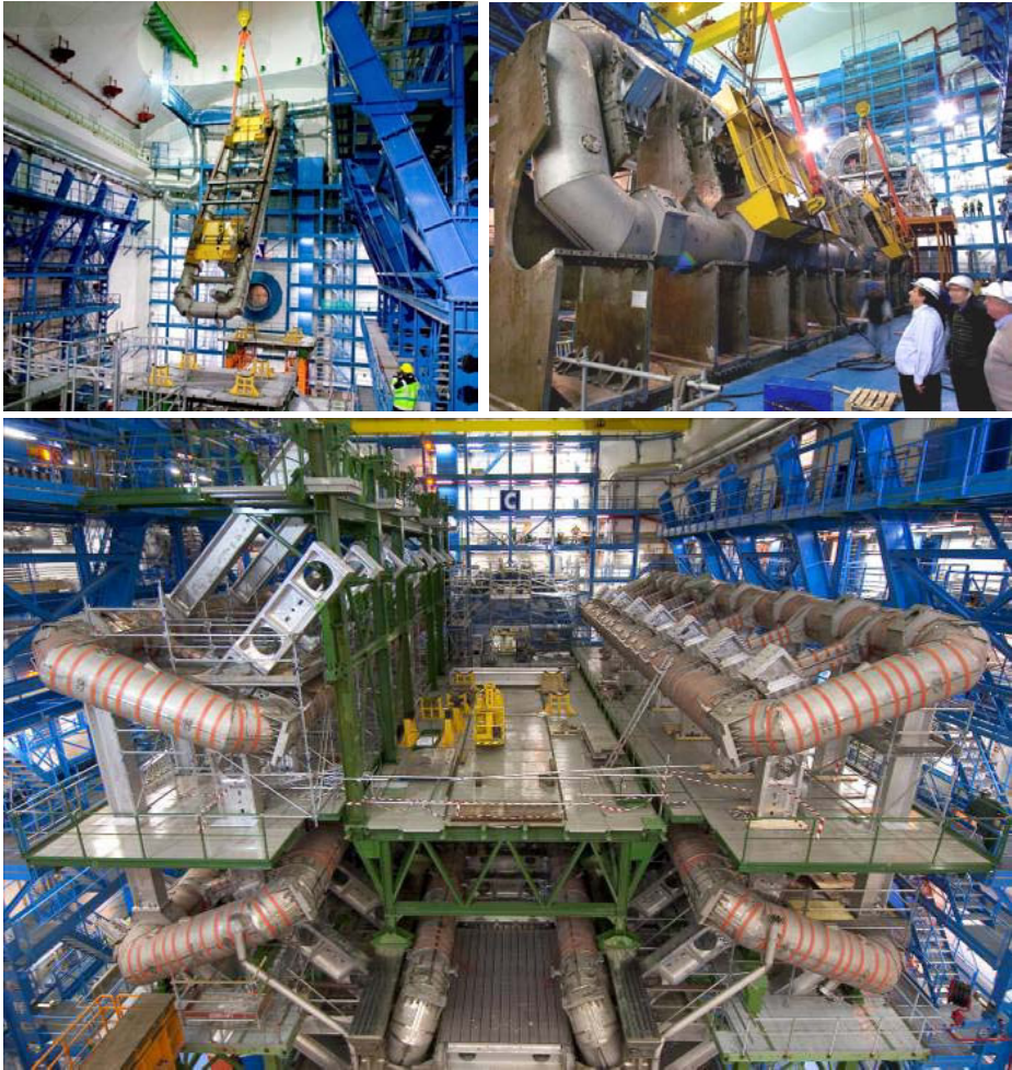
Fig. 11. Assembly of the barrel toroid in the ATLAS cavern: arrival of a BT coil in the cavern while hanging on the crane hook (upper left); manipulation of a 100-ton coil with mm precision during the insertion in the toroid structure (upper right); assembly status after six coils are installed (bottom). Note the various supporting platforms and pillars for keeping the coils in their calculated positions during the assembly.
