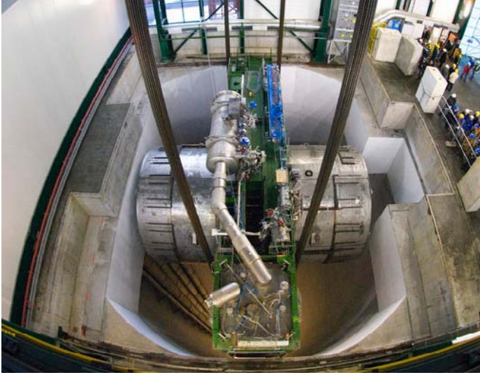
Fig. 3. View of the coil supported from the central section of the barrel yoke, a 2000-ton load, being lowered in the experimental area by heavy lifting means through the 15\text{ m} \times 21\text{ m} shaft opening. It took 10 h to reach the destination 100 m below.
