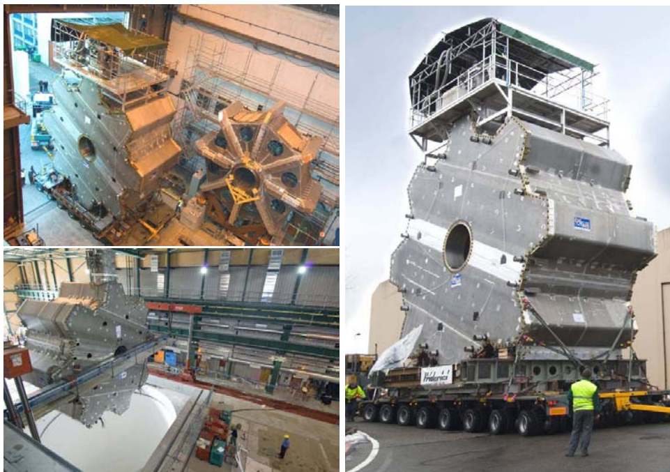
Fig. 13. End-cap toroids on the move: leaving the integration facility (upper left); 240 tons on the trailer to ATLAS point 1 (right), and insertion in the shaft (lower left).
